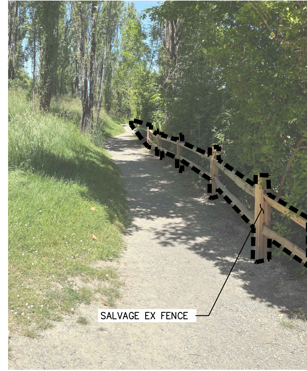
P1 PHOTO NORTH FENCE DEMOLITION
